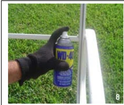
We recommend spaying all bolts with any penetrating oil (WD 40) one hour before removing them. (Pic.8)
